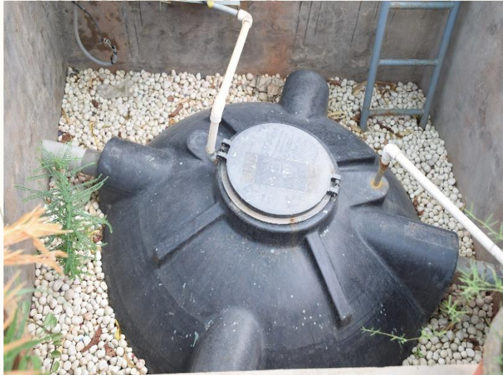
Package Type Sewage Treatment Unit , in plant premises
